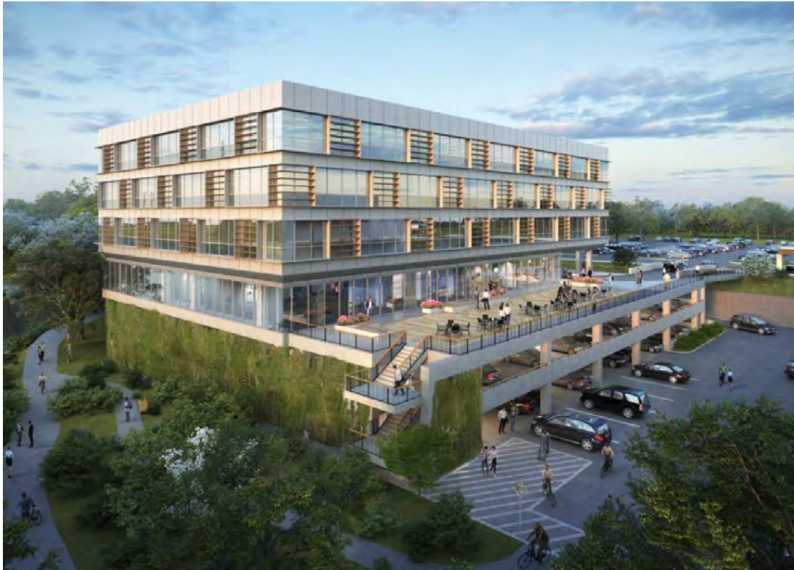
Aerial View from Northeast
